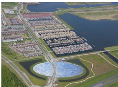
District Heating - Almere, NL
