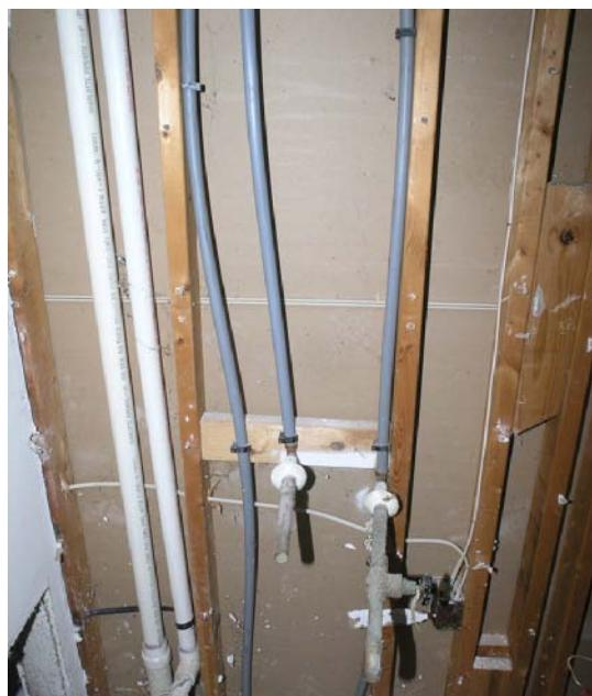
Figure 1. Typical layout of PB piping in a first floor apartment.
