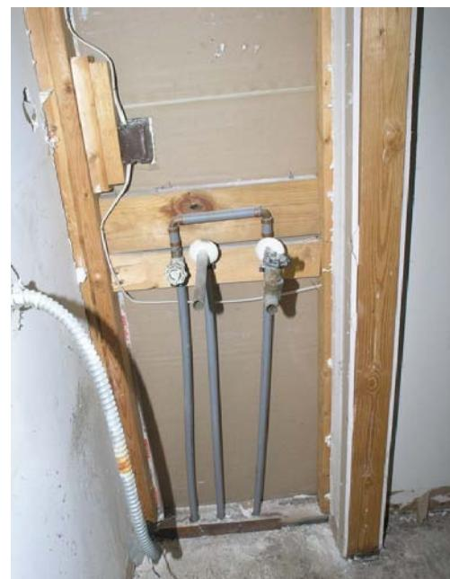
Figure 2. Typical layout of PB piping in a second floor apartment.
